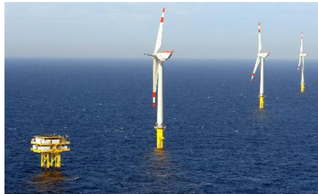
75 MVA 115 / 31 kV hermetic transformer with vacuum tap changer and MS3000 monitoring system for off-shore wind farm Alpha Ventus in operation since 2008
