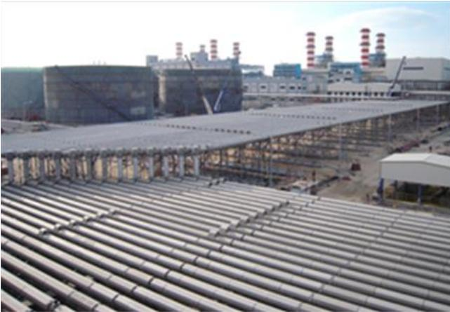
Figure 7. 420 kV Gas Insulated Lines.
