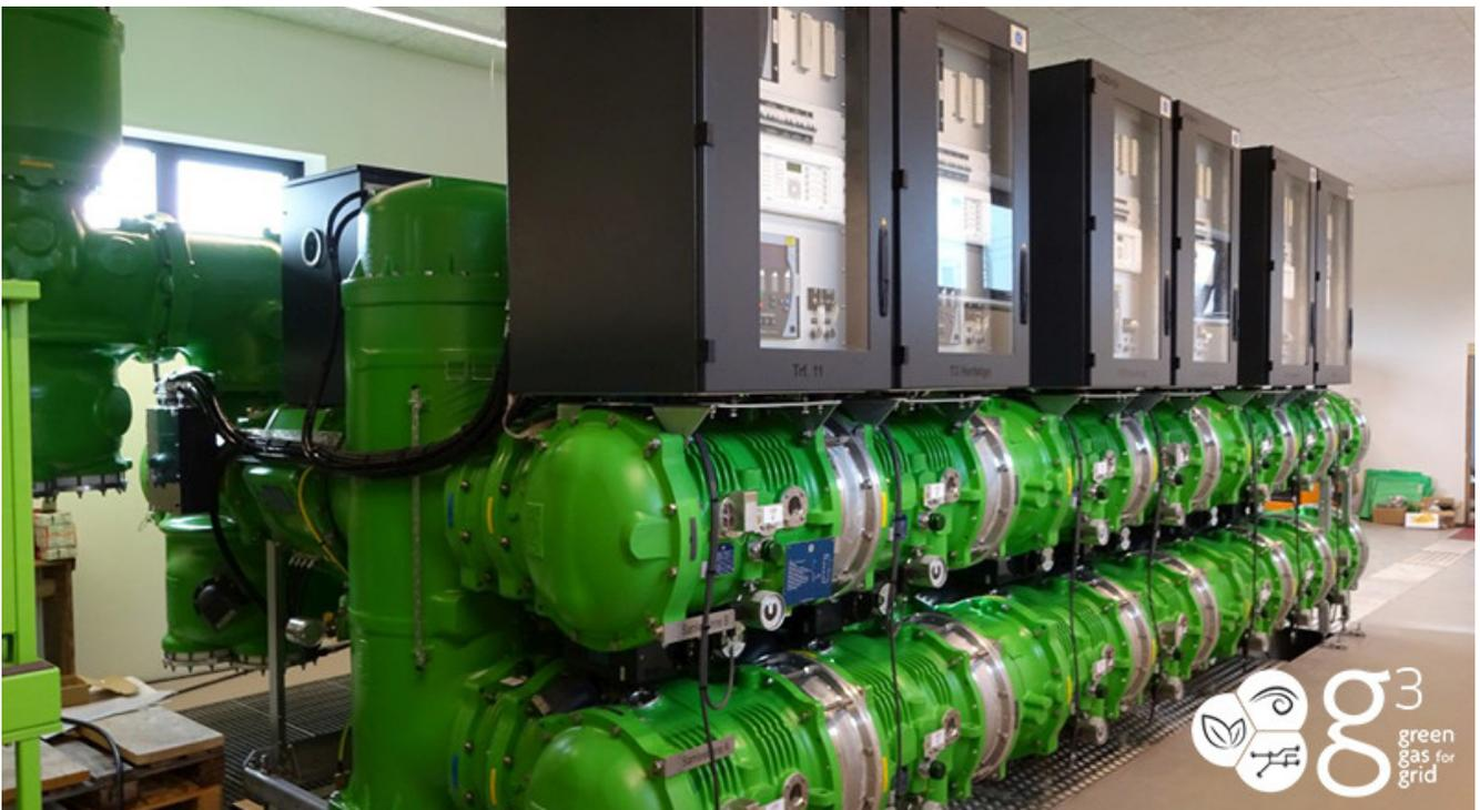
*This Danish SF<sub>6</sub>-free substation, using g<sup>3</sup>, has just been installed in Haslev. Over the next months the bays will be successively energized*
